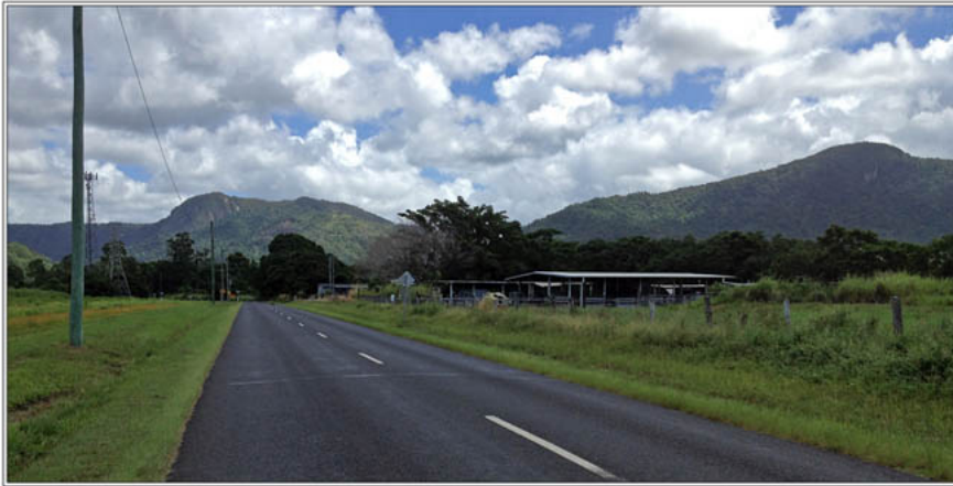
Looking Westwards Along Lower Freshwater Rd
