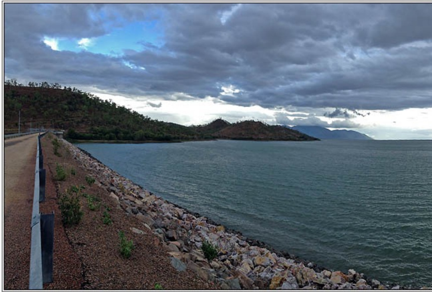
Ross River Dam near the Spillway
